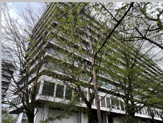
Photo 5: Façade route de Ferney
