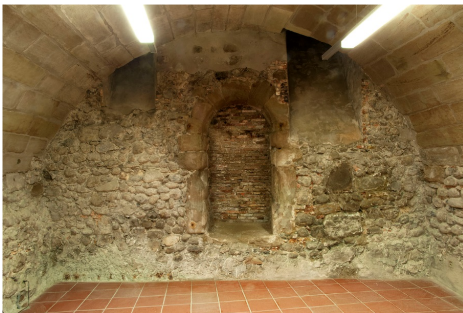
Figure 13. Le mur M 1.
