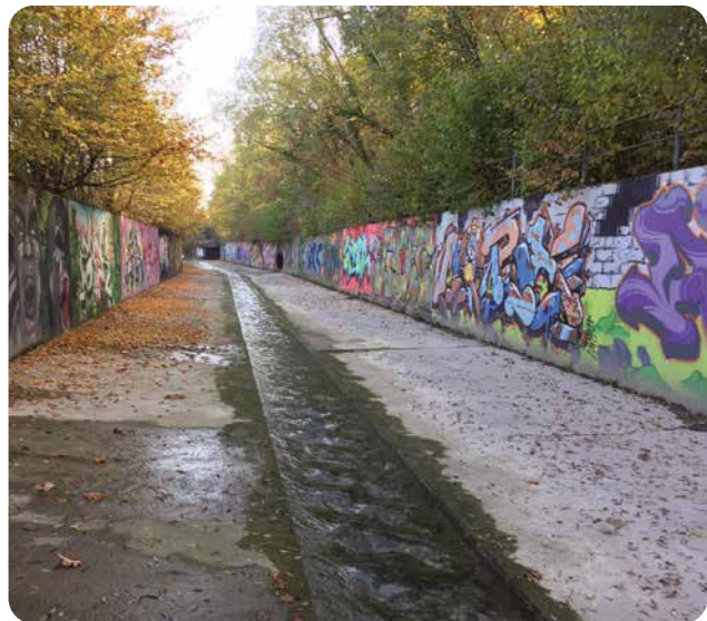
Artificial reach of the Nant d’Avril stream, below the ZIMEYSA industrial area.
