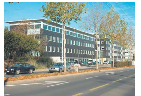
Onex - route de Chancy, Office cantonal de la population.
